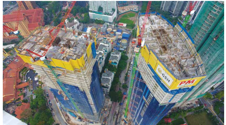
Construction work in progress for Conlay 301 (left) and Eaton Residences (right), both located at KLCC.
