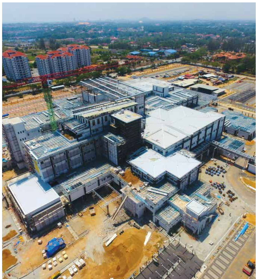
Construction work in progress at UniSZA Teaching Hospital in Terengganu.
