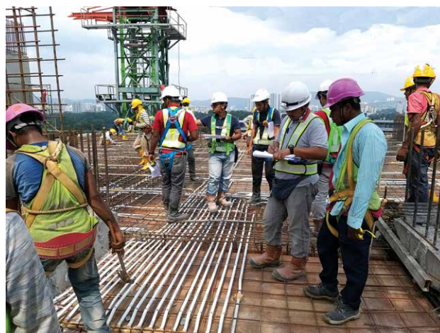
Quality inspection at the Conlay 301 project site.
