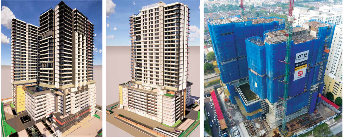
Building Information Modelling of Lot 15, SJCC and the actual construction work in progress at site.
