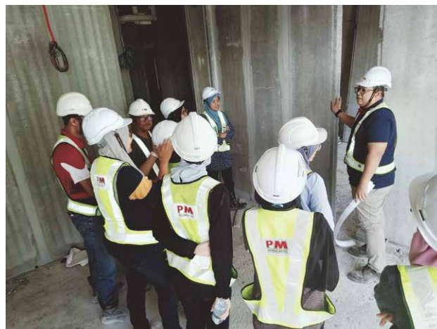
Monthly QA/QC Meeting and Briefing on Lightweight panel tile marble installation at the Eaton Residences project site.
