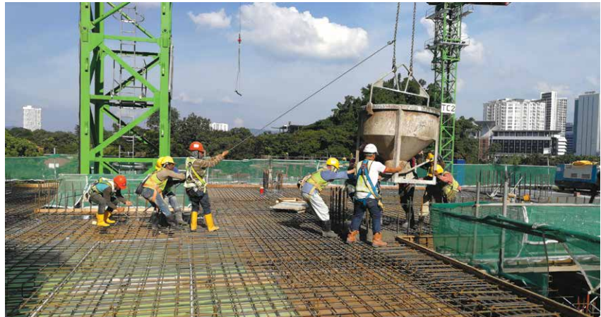
A typical concrete casting in progress at project site.
