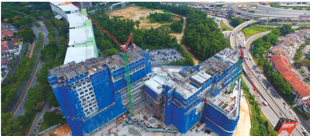
Construction work in progress at Ativo Suites, Damansara Avenue, Selangor.
