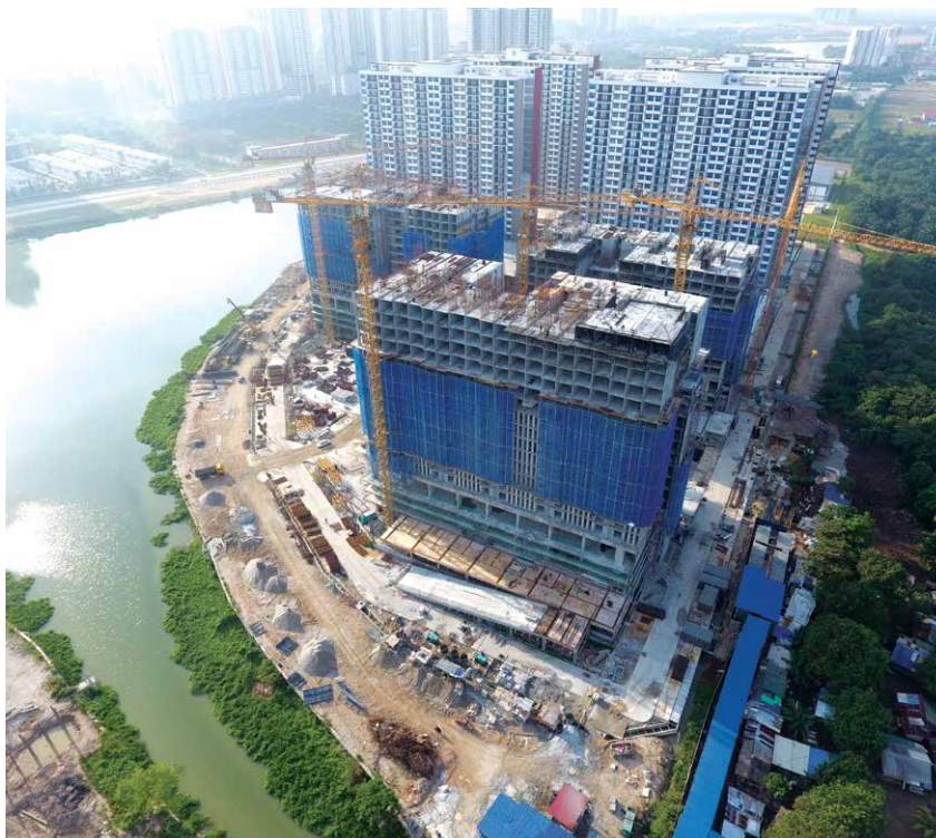
Construction work in progress at LakeFront Homes, Cyberjaya.
