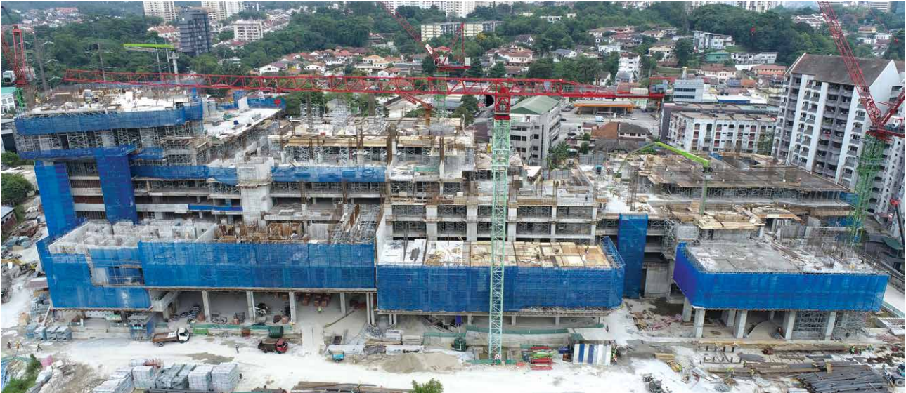
Construction work in progress at TRIA Seputeh in Kuala Lumpur.
