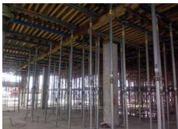
DOKA System which served as foundational support for all high-rise buildings
